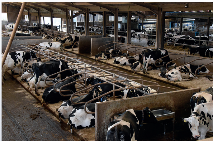
The cubicle shed is fitted with auto-scrapers and LED lighting.
